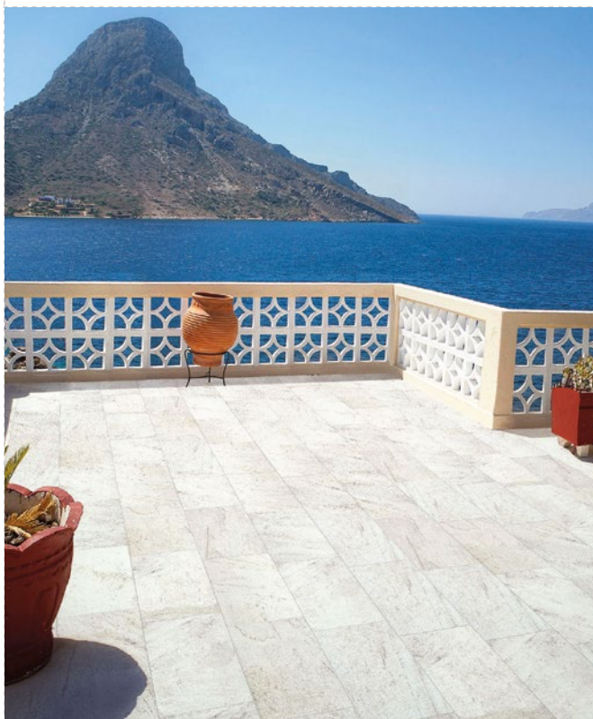
Laying made by: Italian Stones Monte Bianco 30x60 Antislip R11
